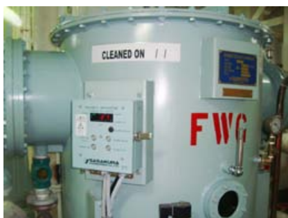
■ Fresh Water Generator having tube type heat
